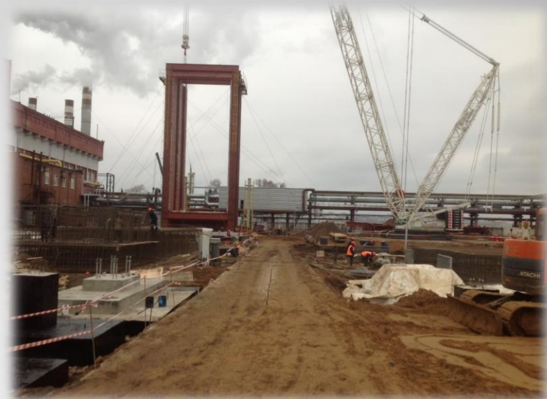
Assembling of boiler-utilizer steel structures
