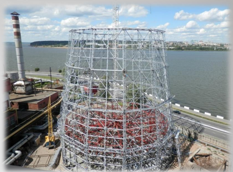
Assembling of cooling tower
