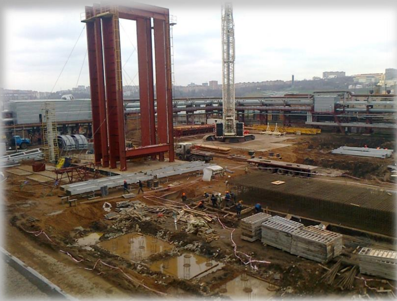
Foundation of gas turbine
