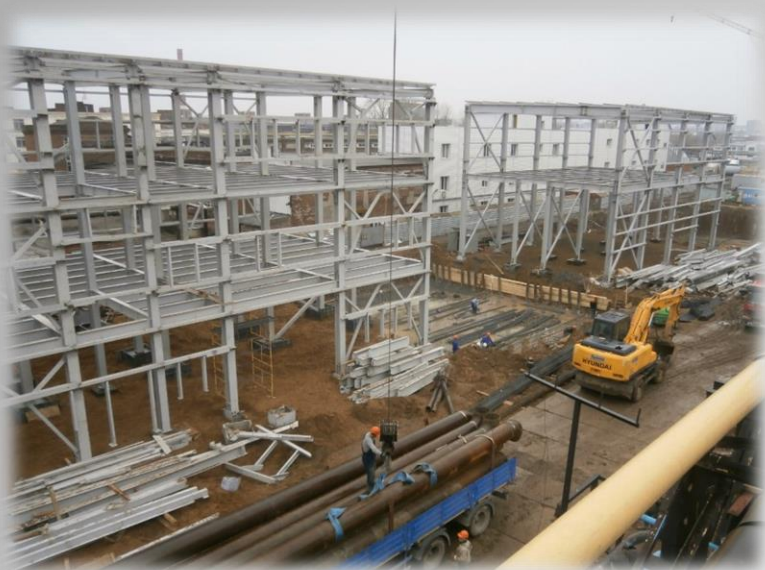
Assembling of main building steel structures
