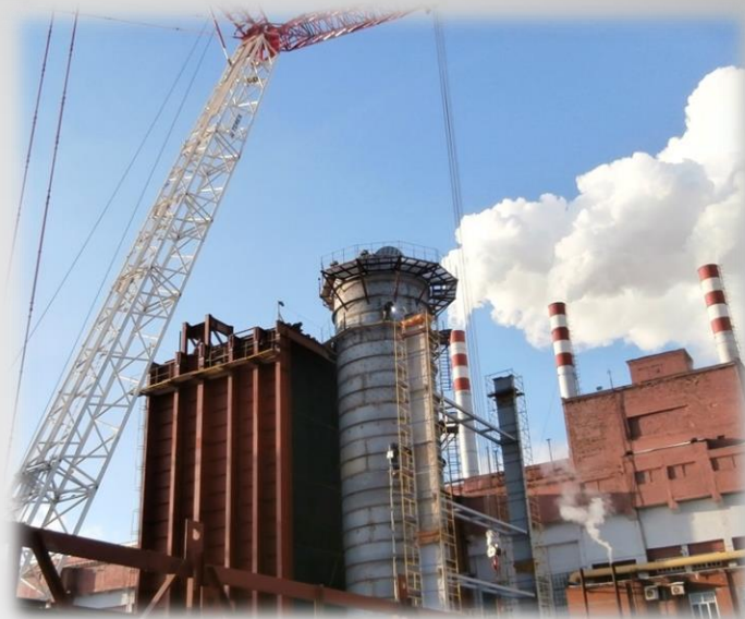
Assembling of flue and boiler-utilizer
