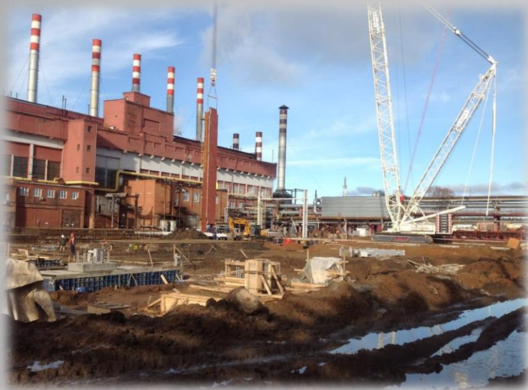
Beginning of boiler-utilizer gas flue steel structures assembling
